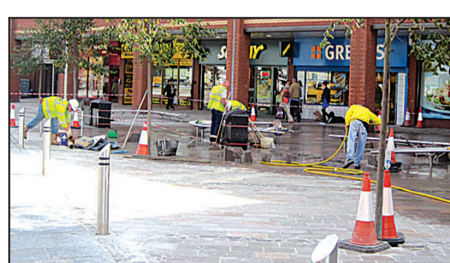
NEW LOOK: Work is completed at the Shopping Centre
