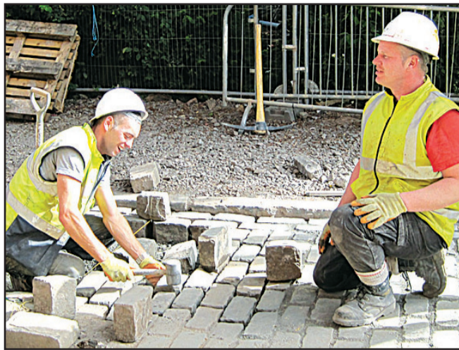
PAVING THE WAY: Workers fit new stone surface at Cross
